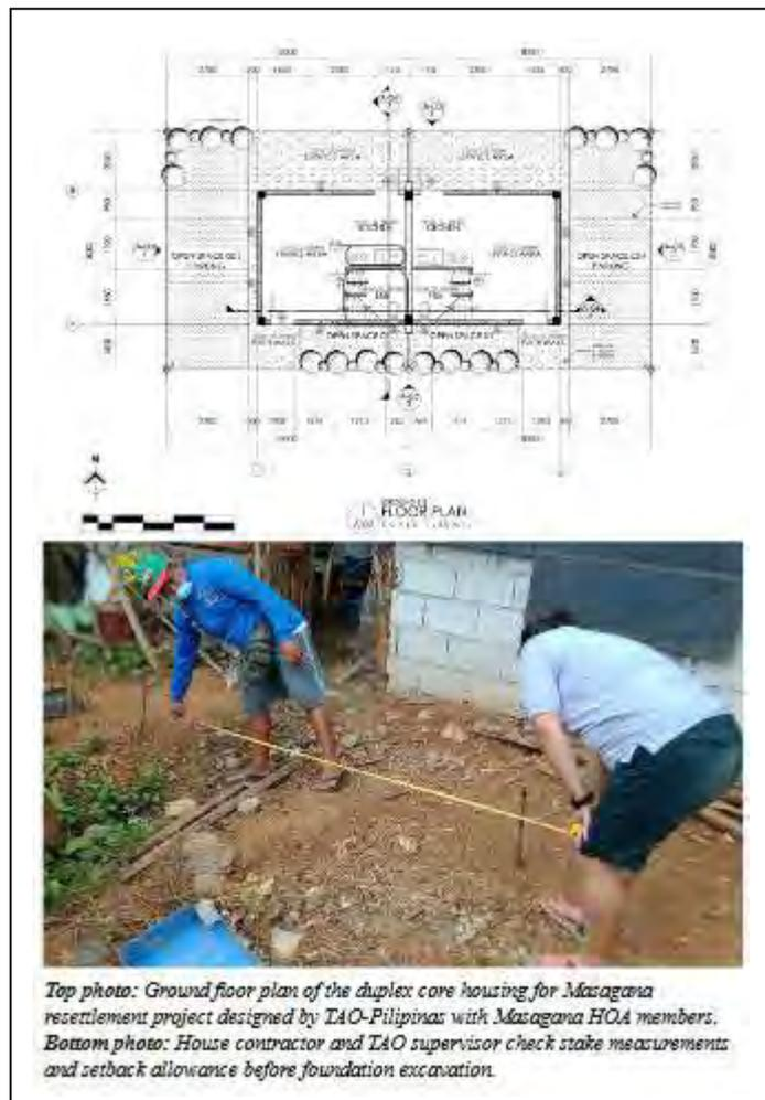
*Top photo: Ground floor plan of the duplex core housing for Masagana resettlement project designed by TAO-Pilipinas with Masagana HOA members. Bottom photo: House contractor and TAO supervisor check stake measurements and setback allowance before foundation excavation.*
